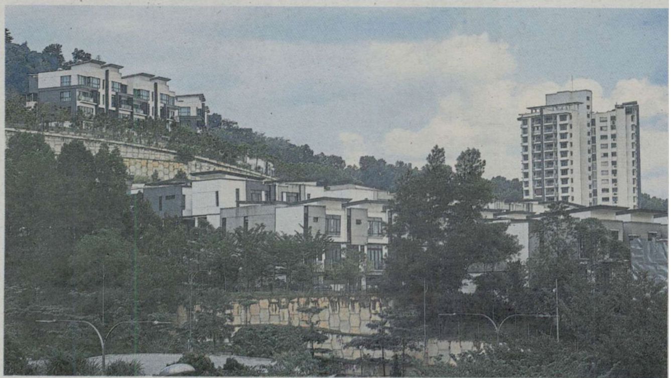
In Malaysia, affordable housing — particularly homes with quality space for the healthy development of families — remains a concern
