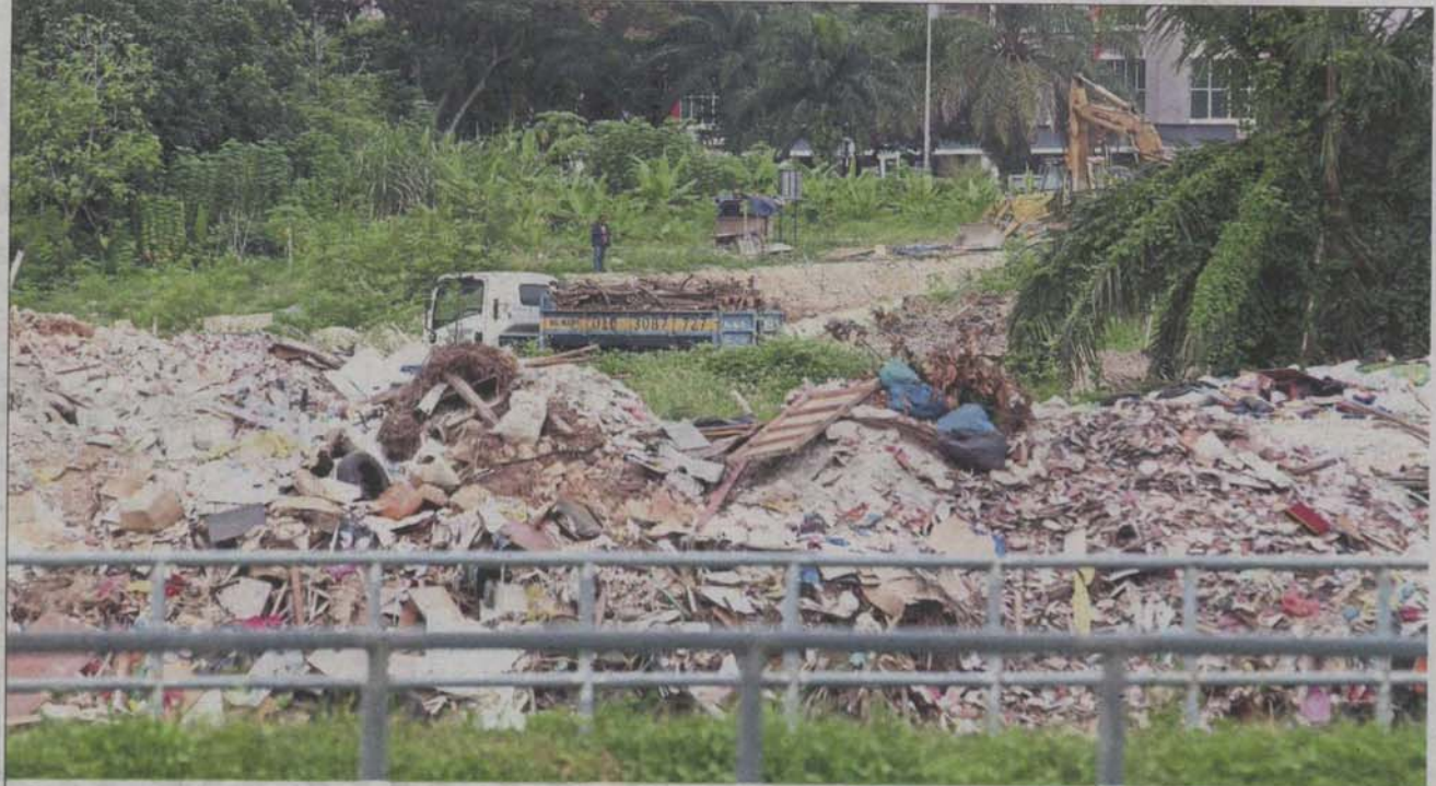
Construction waste which is often discarded is an untapped resource. — Filepic
