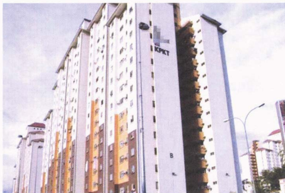
RM100 mil for the repair and refurbishment of low- and medium-cost strata housing is considered inadequate
